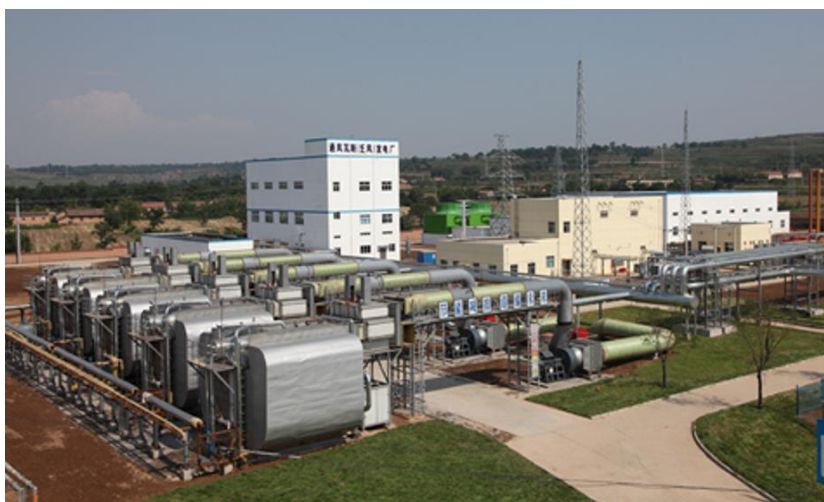
Figure A-III 9: Ten RTO units at the Dafosi mine (Courtesy of CCII)
