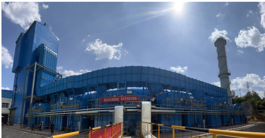
Figure A-III 6: Six Twin bed RTOs at a Shanxi mine (Courtesy of Anguil Environmental)
