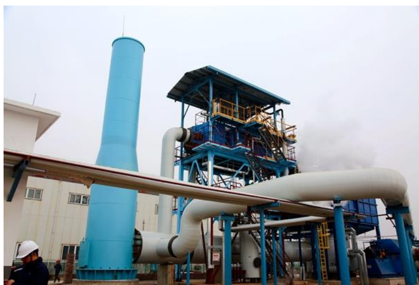
Figure A-III 10: VAM RTO of Yiyang Clean Energy of Zhejiang Province (Courtesy of CCII)
