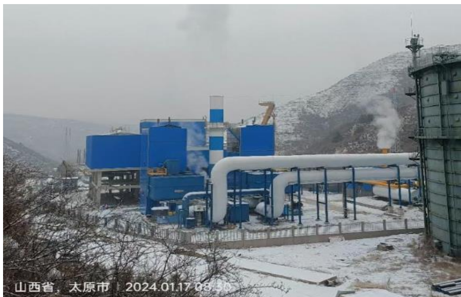
Figure A-III 8: Two Rotary RTOs at the YuangXiang coal mine (Courtesy of Eisenmann Environmental Technology)
