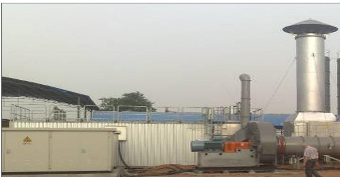
Figure A-III 2: Single bed RTO installation at GaoCheng mine (Courtesy of MEGTEC-Dürr)
