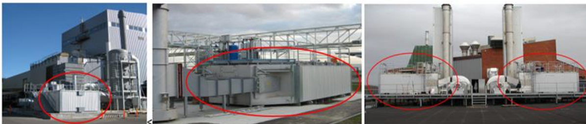
Figure A-II 2: Industrial installations of single bed RTOs (Courtesy of MEGTEC-Dürr)
