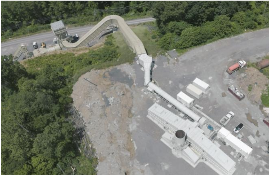
Figure A-III 7: Large Twin bed RTO at Buchanan mine (Courtesy of Biothermica)
